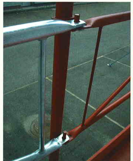
Alu and steel scaffolding can be mixed together
